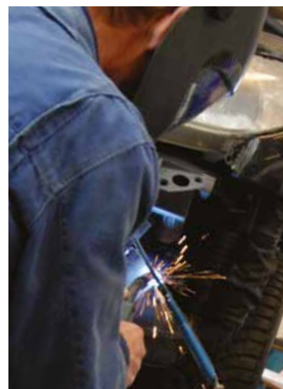
MIG brazing maintains the strength of the steel and protects the anti-corrosive zinc surface
